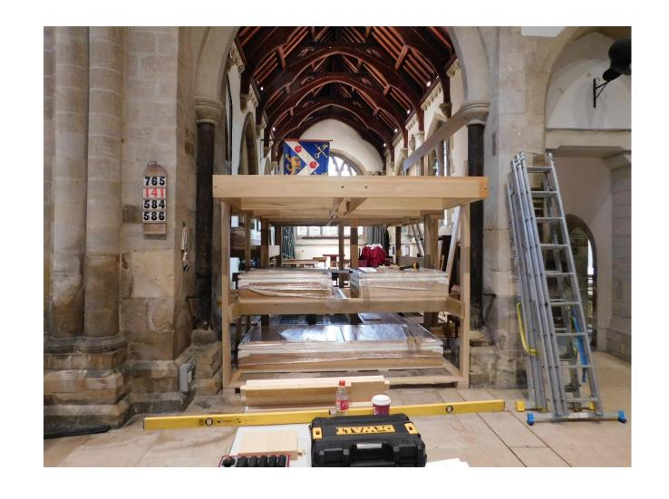
A new platform was constructed over the passageway to provide extra space for pedal stops and the 32ft pedal pipes which now form part of the back of the case facing into Trinity Chapel.
