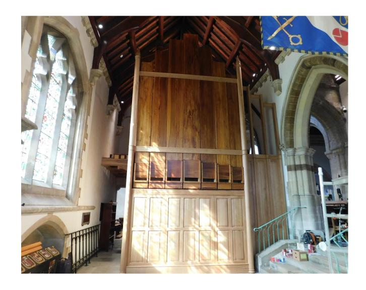
The new Swell box was erected in a more forward position than previously and the picture shows the view from the Nave through to the new rear shutters and pedal pipes beyond
